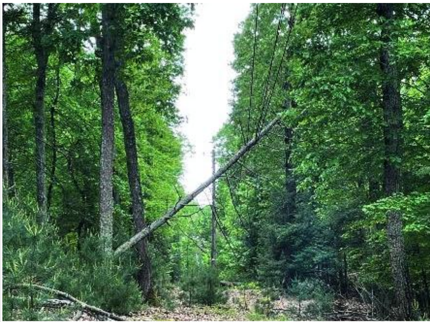
Immediate EFD detection and location of a vegetation strike on covered conductors
